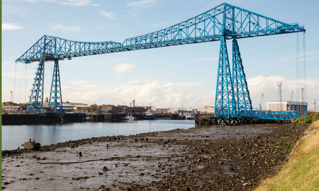
Transporter Bridge, Middlesbrough, UK
