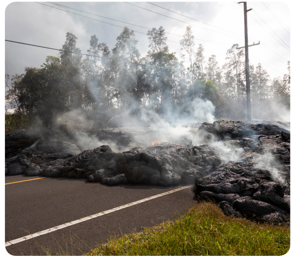
Road in Hawaii destroyed by lava
